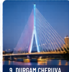
9. DURGAM CHERUVA CABLE BRIDGE
